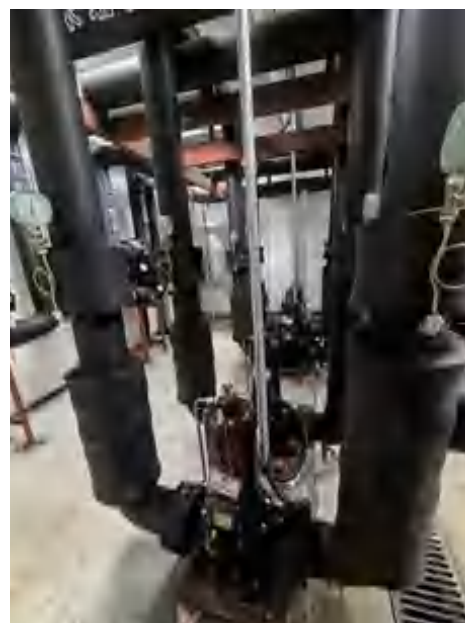
Replace the water pump in the computer room and install shock-absorbing pads
